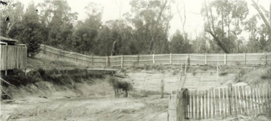
1908 - Pool under construction
